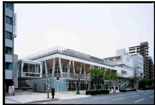
Hakata Elementary School, Naraya Community Center 2001, Kazumi Kudo + Hiroshi Horiba / Coelacanth K&H Architects Inc. ©SHINKENCHIKU-SHA
